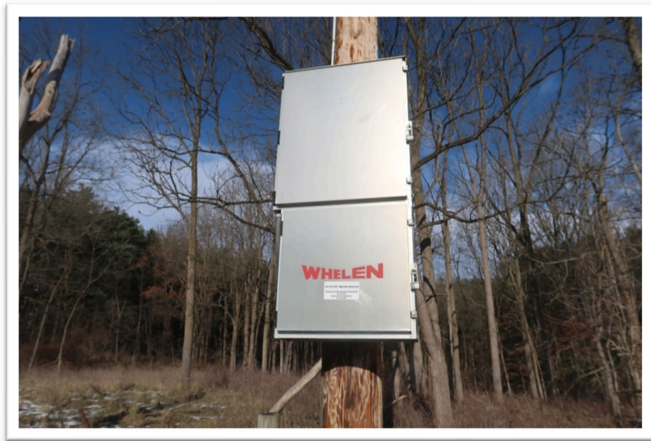
Photograph 19: Typical view of Whelen emergency siren controller
