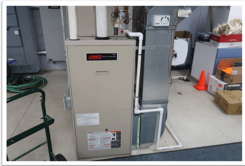
Photograph 11: Typical view of Dexter Township Hall forced-air furnace
