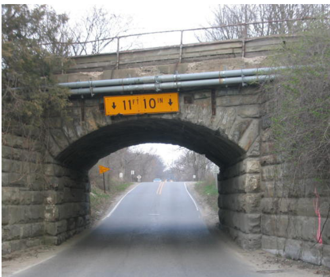
Island Lake Road Norfolk Southern rail underpass
