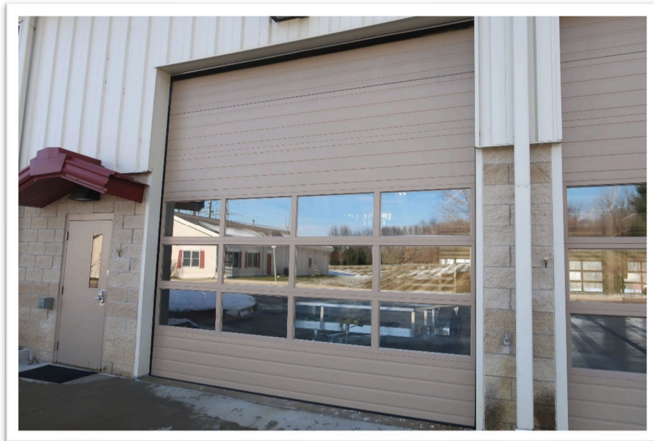
Photograph 16: Typical view of Dexter Area Fire Department overhead door
