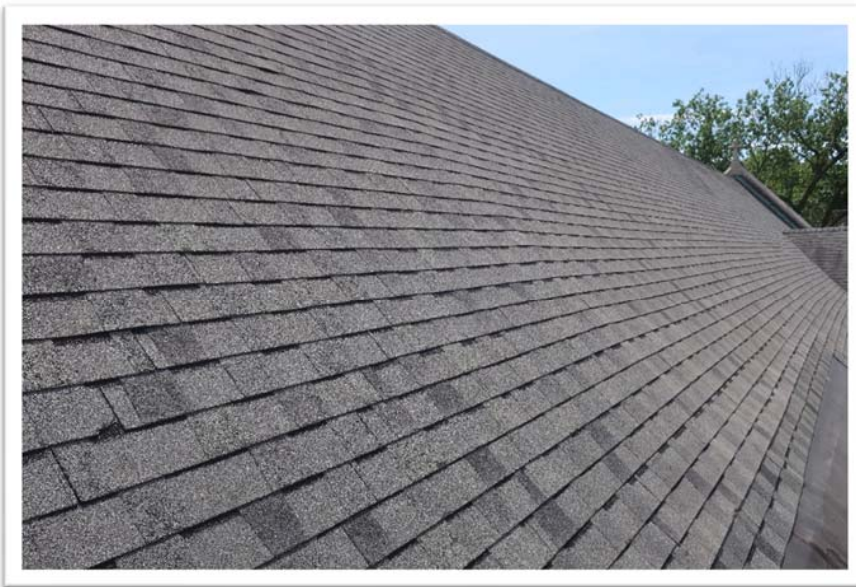
Photograph 14: Typical view of sanctuary asphalt shingle roof
