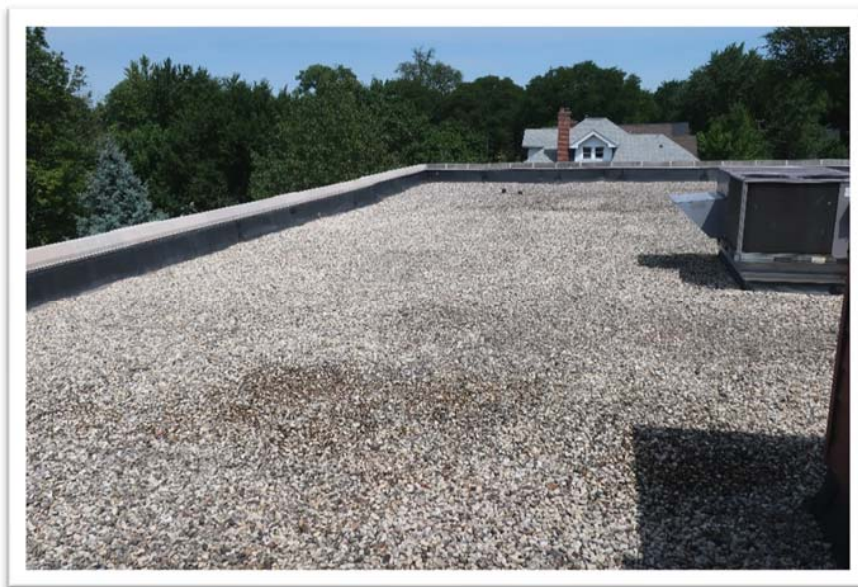
Photograph 16: Typical view of Kensington EPDM roof
