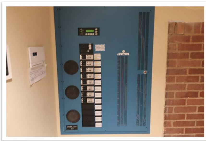
Photograph 30: Typical view of sanctuary master light panel
