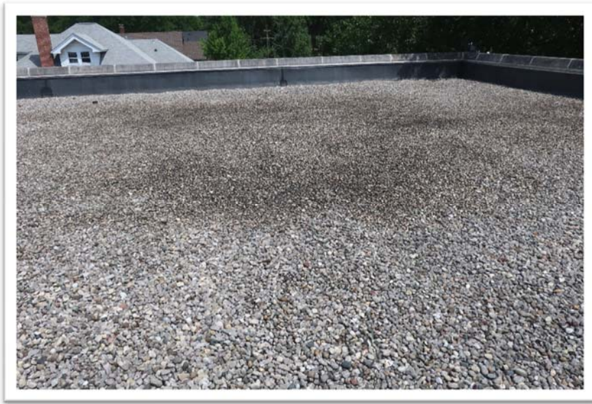
Photograph 17: Typical view of Kensington EPDM roof
