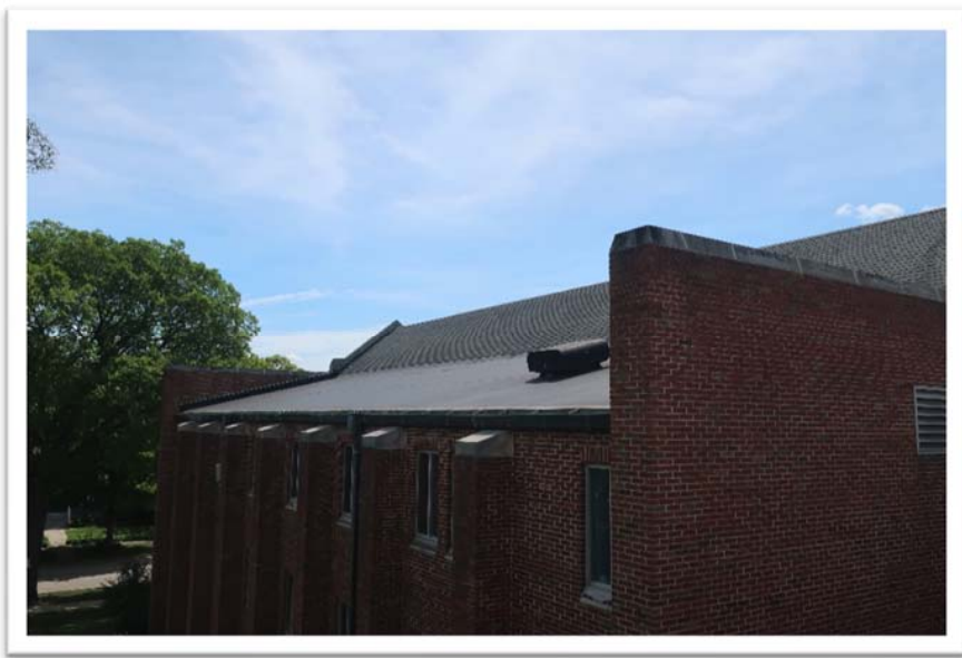
Photograph 18: Typical view of Catherine roof (EPDM and asphalt shingles)
