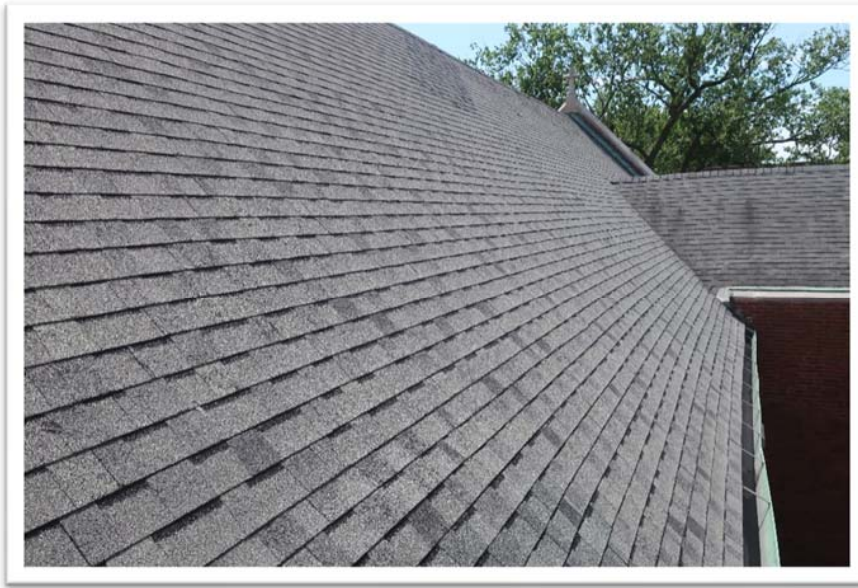
Photograph 15: Typical view of sanctuary asphalt shingle roof
